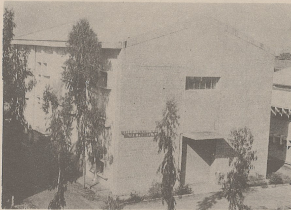
(a) Water Tunnel Building
