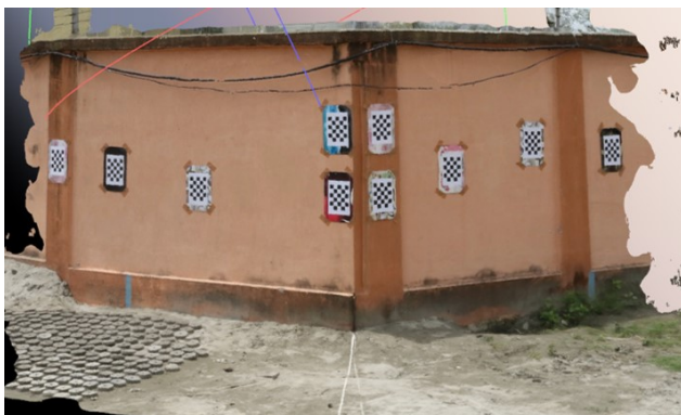
Figure 8: 3D mesh model of 55° corner
