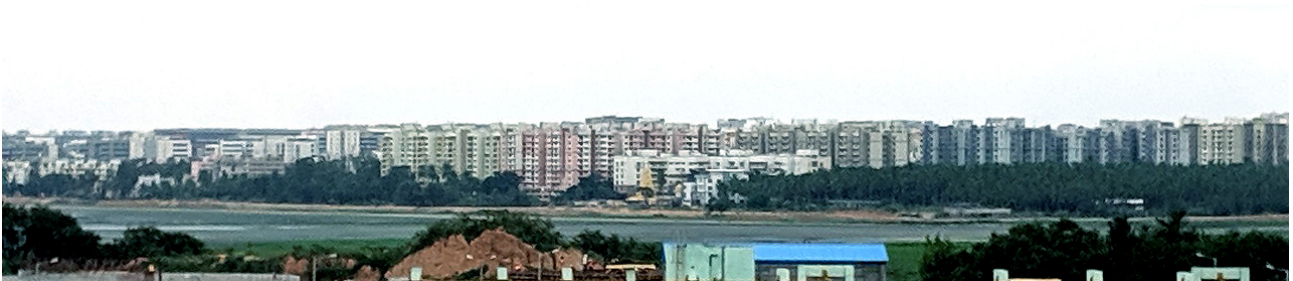
Figure 1: Bellandur Lake skyline showing some of the most intensely populated and built up area. The view shows about a quarter of the shoreline only. At this time the water of the lake in the foreground is drained to clean it up.
