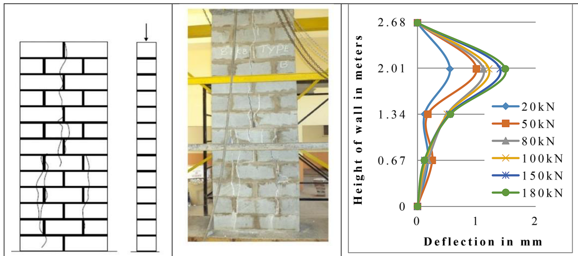
Fig. 6 Views of failure patterns and distribution of lateral deflection along the height at various stages of loading of wall no. 2 (HCB-200-A2)
